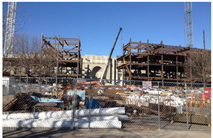
Construction around Memorial Stadium outside Oldfather.
