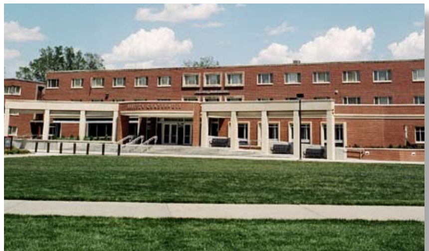
Selleck Quad renovation, 2004
